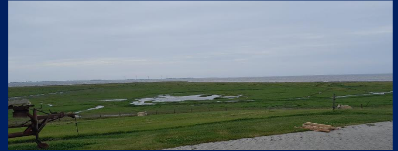
Pipe fills during an upcoming land-under
